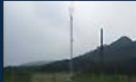
Automated Synoptic Observing System(AWS)
